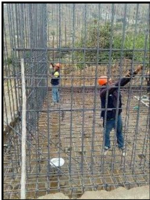
The beginnings of the new reservoir in Samne, Peru!
